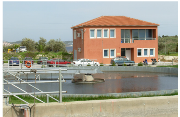
Secondary clarifier and administration building at the Mytilene STP
